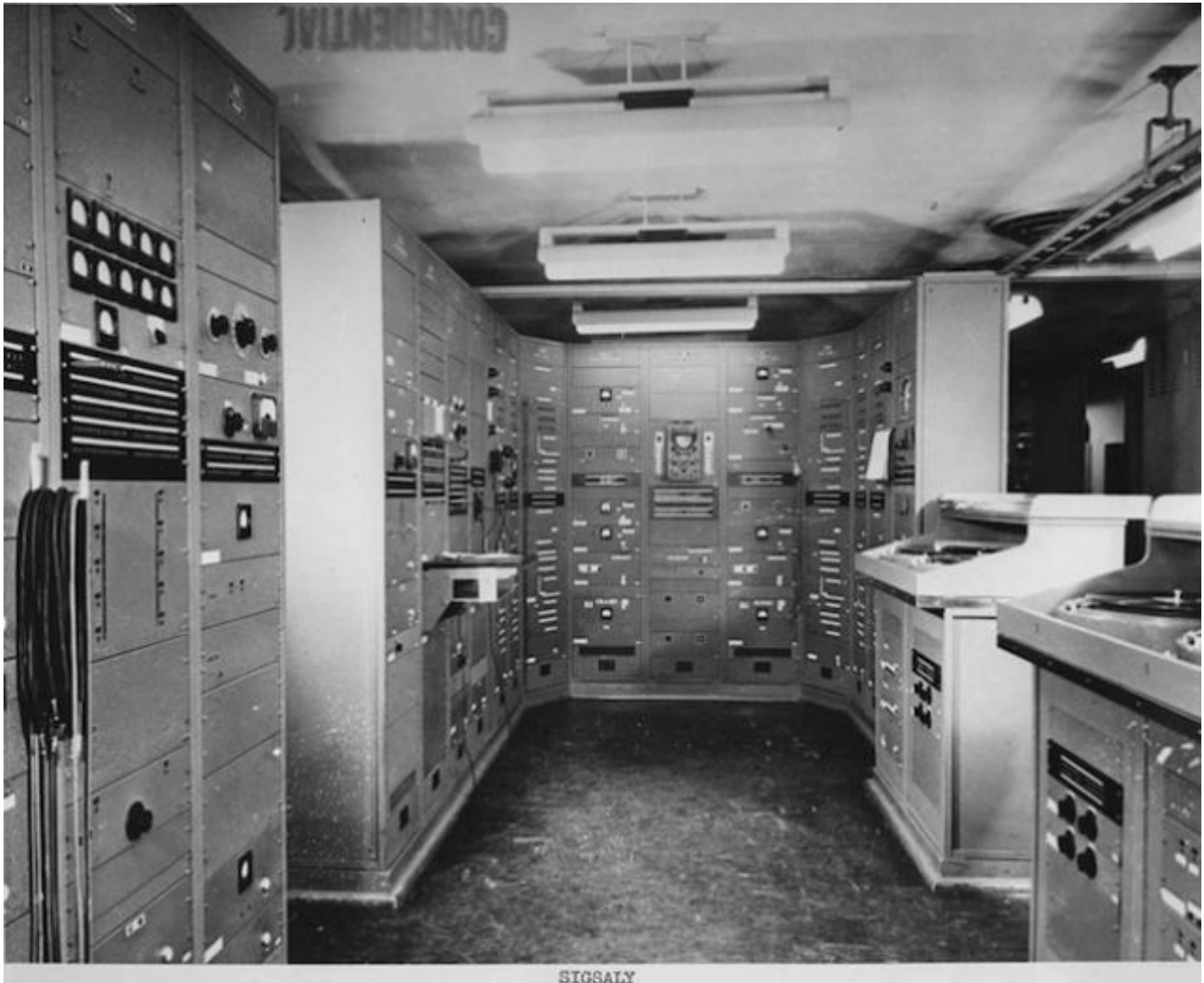
Fig. 10. SIGSALY equipment in service during World War II
